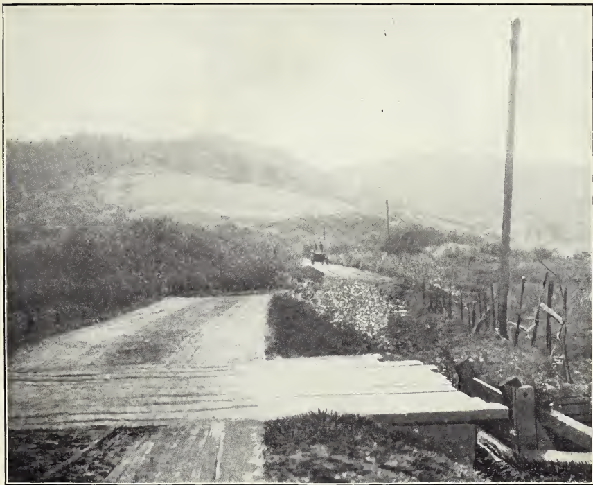
A. ROAD CROSSING FAULT TRACE NEAR POINT REYES STATION. Looking southwest. Offset, 20 feet. Photograph by G. K. Gilbert.
